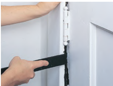
1 Carefully remove and save interior trim
