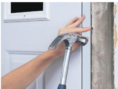
4 Nail replacement unit into position
