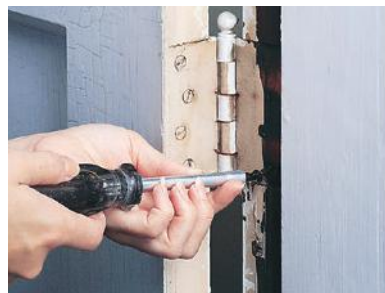
2 Remove the old door, strike plates, hinges and threshold
