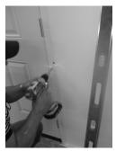
3. Install the remaining screws in the hinge jamb starting at top, checking for plumb as you work toward the bottom.
