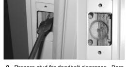
**9.** Prepare stud for deadbolt clearance. Bore a 7/8"-1" hole to a depth of 1" from rabbet of frame. Drill a 3/8" dia. hole at each corner to a depth of 1" from rabbet of frame.
