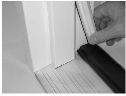
**12.** Pull weather-strip out of the kerf near sill to allow room for caulking. Install sill extender if required.
