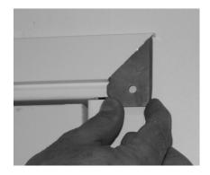
3. Insert casing corner brackets into header.
