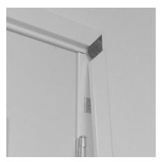
**4.** Slide jamb casing over corner bracket. Push casing upward to meet miter on header casing. Adjust header casing and jamb casing to obtain a tight miter joint. Position casing over outside edge of clips and tap casing toward inside of frame near each clip to snap it over clips. Repeat for other jamb.
